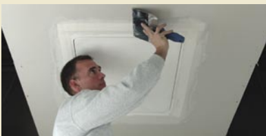
4. Tape and apply drywall compound.
