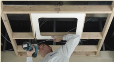
2. Mount Stealth surround with drywall screws.
